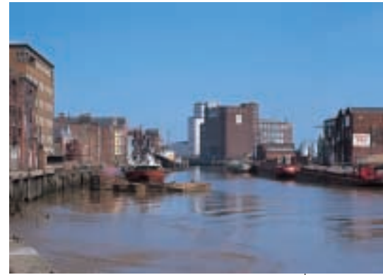
A new pedestrian swing bridge will span the River Hull connecting visitors to the heart of the city's Old Town quarter Photograph courtesy of Michael Palframan
