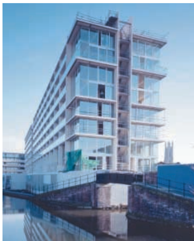
Timber Wharf under construction
