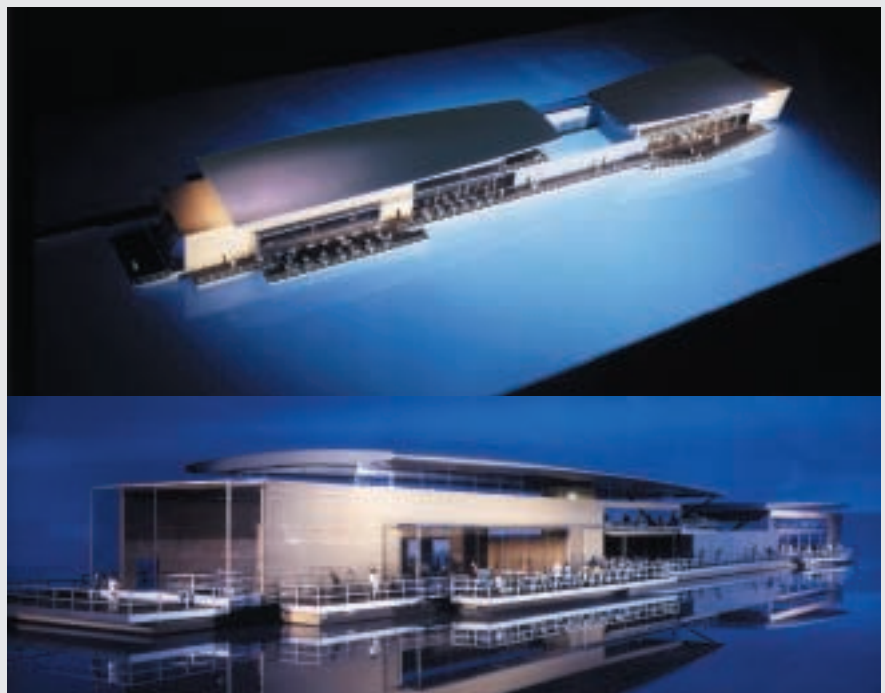
Offshore's structure will sit low in the water with two storeys above the waterline and one below Image courtesy of Koetter, Kim & Associates (UK)
