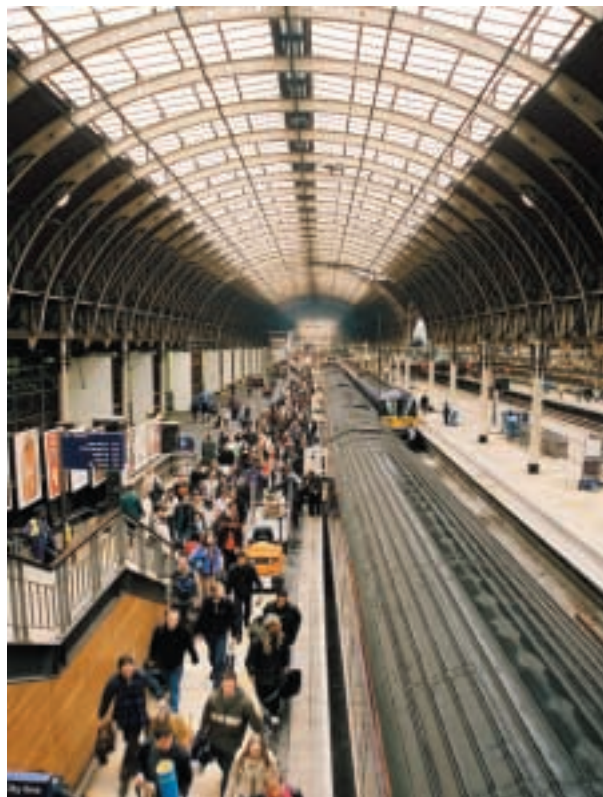
Paddington Station roof
