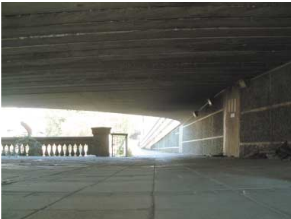
Concrete Jungle, Brent Cross Underpass
