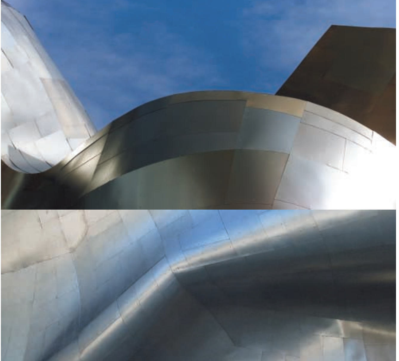
Over 21,000 aluminium and stainless steel shingles cover EMP's exterior Picture courtesy of Stan Smith
